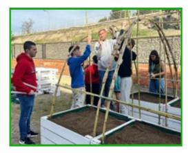
Once the structure was finished, we covered it with greenhouse plastic. We stapled the plastic to the outer walls of the big wooden fruit boxes and screwed a wooden slat on it to reinforce the joint.
