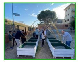
Finally, we reinforced the cane structure with horizontal cross beams and interior pillars also made of cane and joined with hemp rope and open pieces of reused irrigation pipe.
